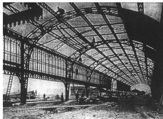
fig.5 perronoverkapping station 's-Hertogenbosch 1896
